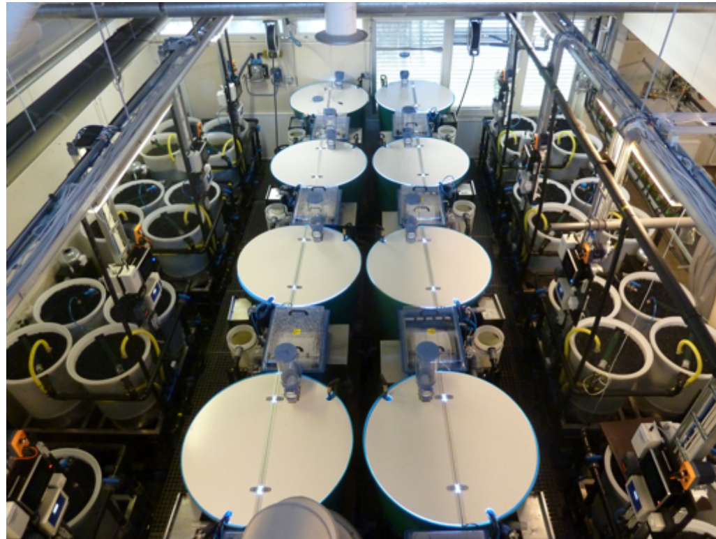
Luke RAS research facility at Laukaa
